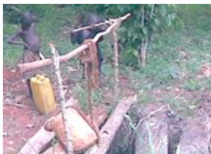
Photo of Curious Kids at the new hand dug well trying out the improvised shadoof system (above)
